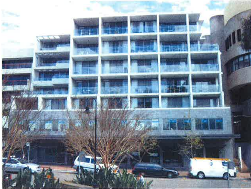
Figure 12 – Mixed use development at 26 Clarke Street
