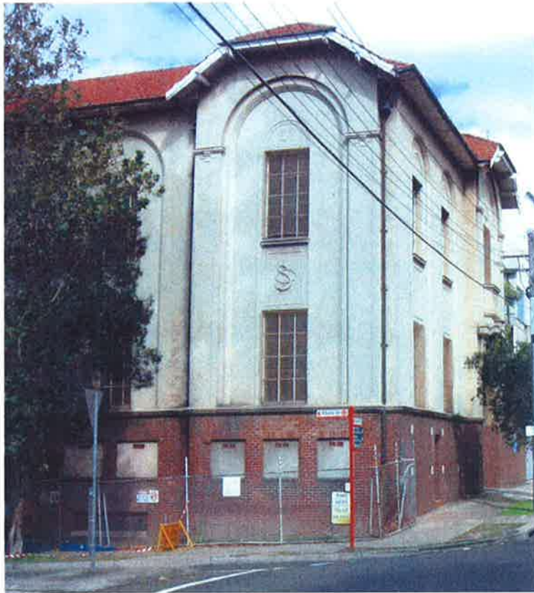
Figure 14 – The heritage listed electricity sub-station
