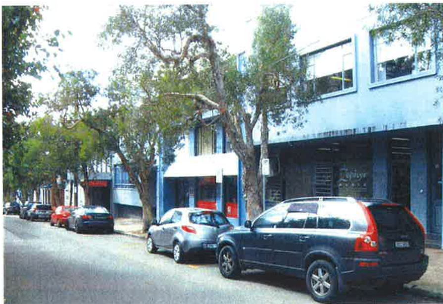
Figure 11 – Aging 2-3 commercial buildings on Hume Street
